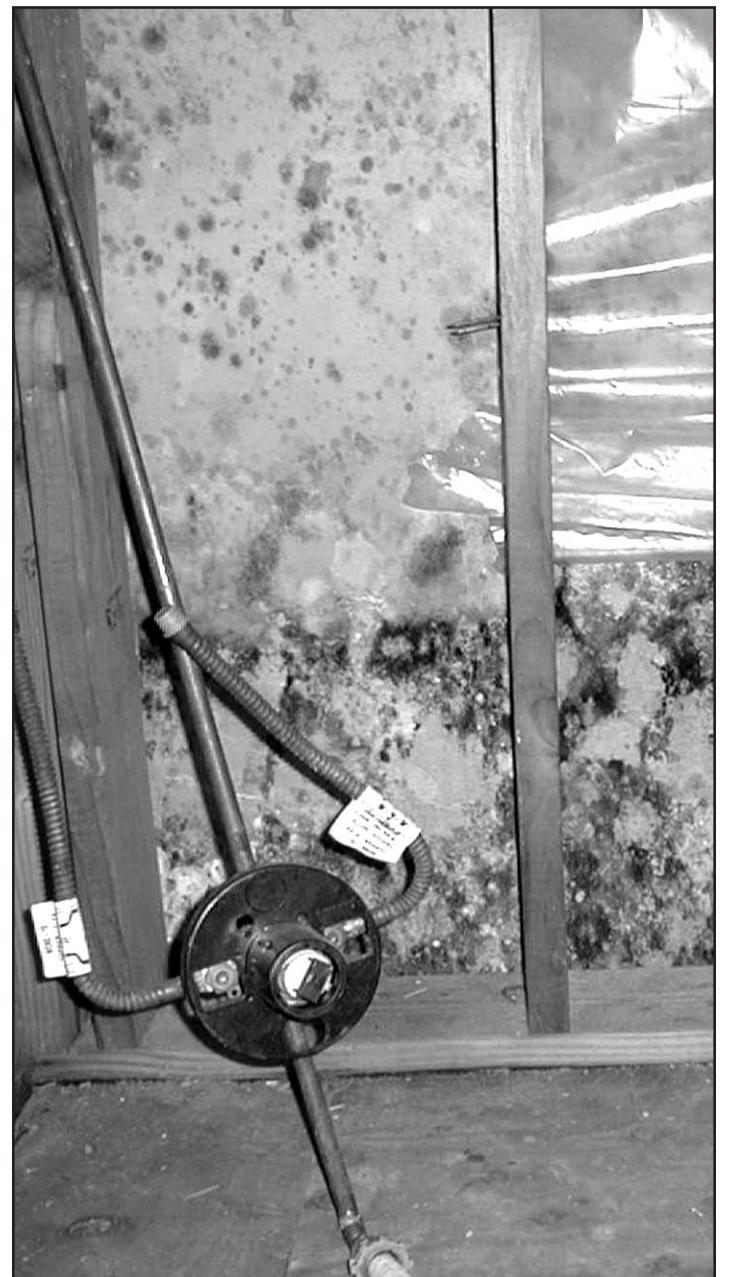
and in wet areas such as showers and basements.
